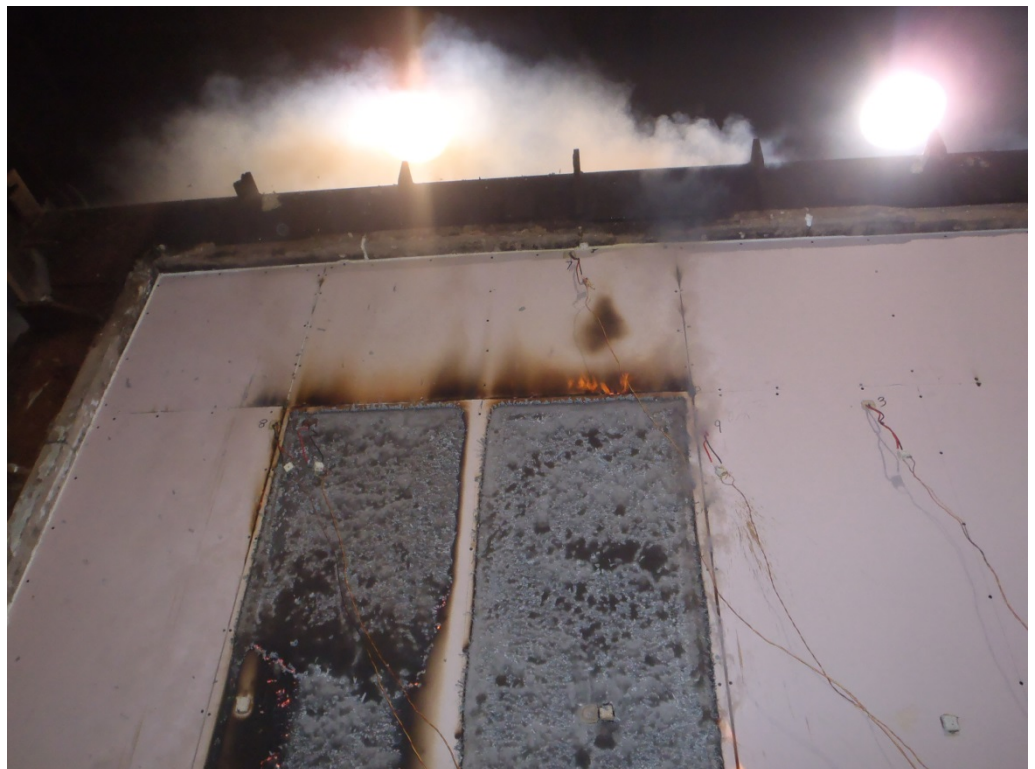
The unexposed face of the test construction after 91 minutes of testing showing the flaming at the joint of the partition.
